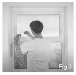
1. Using a credit card as a guide slot a bracket into the corner of each gasket seal on the bottom window. (Fig.1) (Fig.2) Repeat for the top window. (Fig.3)
